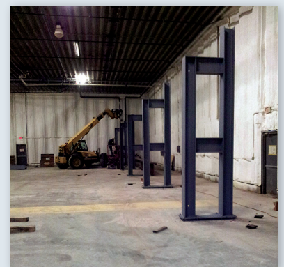
Erected crane columns
