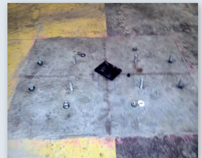
Crane column pile caps poured flush with slab
