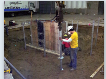
Advancing helical pile lead section
