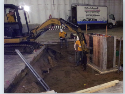
Helical pile installation for equipment mat foundation
