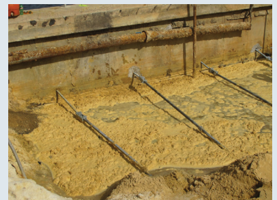
Helical tiebacks with threaded rod extending through seawall; prior to pre-tensioning
