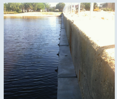
Waler system on stabilized seawall
