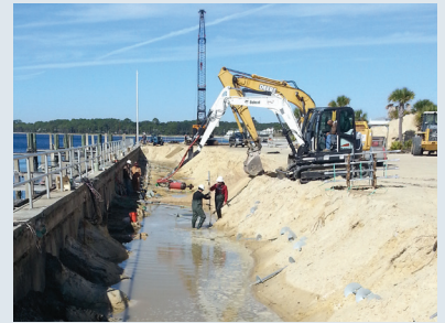
Excavation made behind seawall for tieback installation
