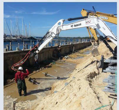
Aligning HA175 lead section for advancement
