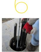
Terminate the helical pile shaft and install the bracket. Ensure bolts are tight and the bearing plate is level and centered.
