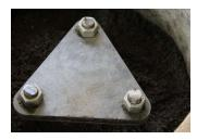
Tighten the nuts against the bearing plate once the structure is lifted or stabilized. Cut rod leaving a minimum of 1/4 inch above the nuts.
